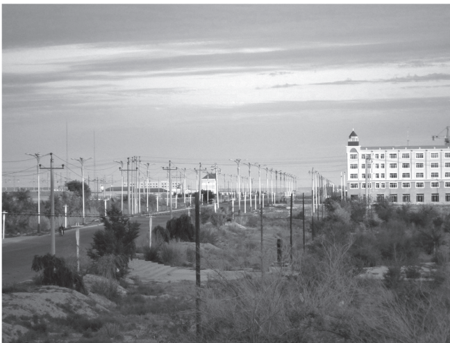
Fig. 10 Wind turbines and the town's electric power station (Ereen city, August 2010). Photo: G. Lacaze.
