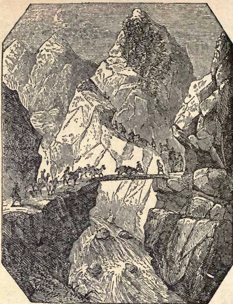
Bridge of Ghamda.
