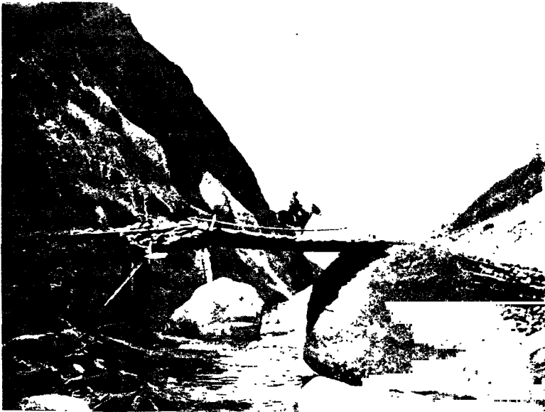
BRIDGE OVER THE GHEZ-DARIA
